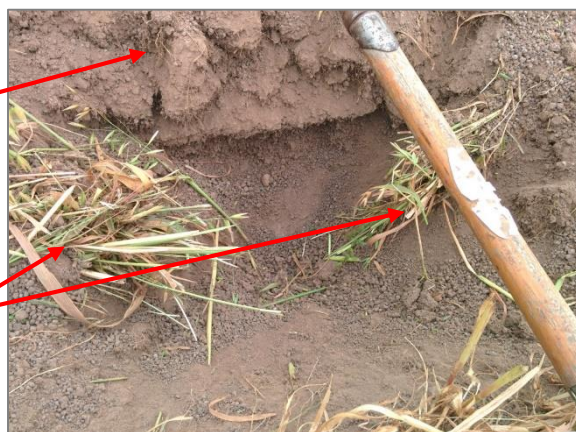
Figure 6: Placement of in-situ harvested material (Image: Domenic Germano)
