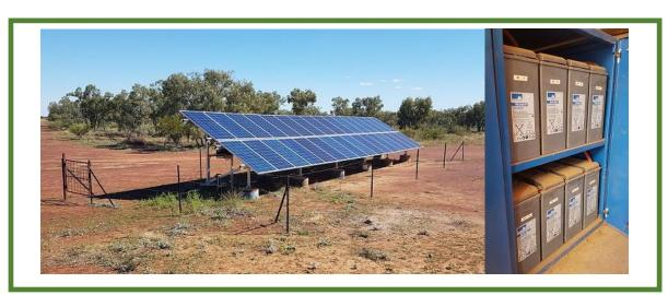
The system comprises 8kW solar panels with 16 batteries providing 16kW of usable batteries. There are two 5kW inverters and a smart system that switches between feeding electricity to the house and then excess to the battery. Similarly, the smart system switches from the panels to the battery to feed the house when the solar panels are not providing enough power to meet the needs of the house.
